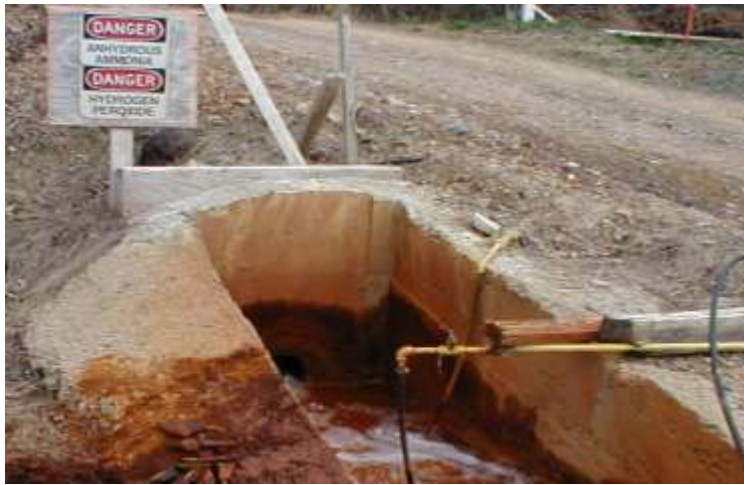
Figure 5: Hydrogen Peroxide Method of Treatment [1]
